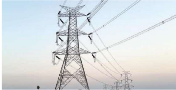
Crucial metric: Reliable electricity is a fundamental enabler of economic and social development.
